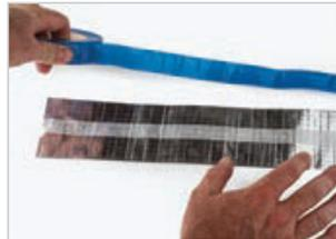
2. Measure the blue strapping needed to go around the duct and back up to the hang point on the roof.
