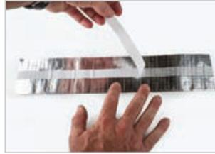
1. Measure the Sisalation to the desired length and peel back the double sided tape backing.
