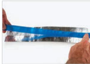
3. Find the halfway point of the blue strapping that you have cut so equal amounts will hang over each end and stick it on the sticky tape on the sisalation
